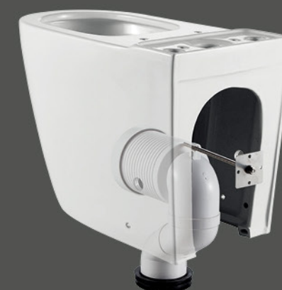
Installation of sewage pipe
